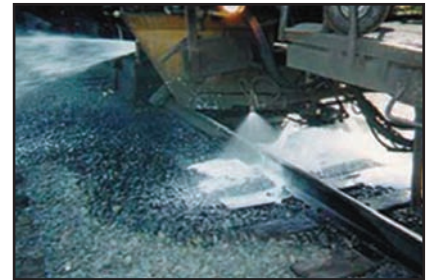
Fire suppression systems include separately controlled wide-angle air injected tie and ditch sprays.
