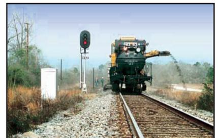
**Ballast discharge.** The HP distributes the cleaned ballast along the shoulders, at a rate that can be varied for local conditions. Plus, it establishes the railroad specified shoulder slope as it works at speeds of up to 2 mph (3.2 kph).
