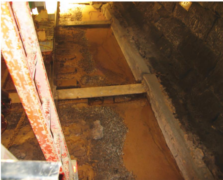
Prior to any work being done in the tunnel, Atlas had to stabilize the walls with crossbeams in order to hold them in place.
