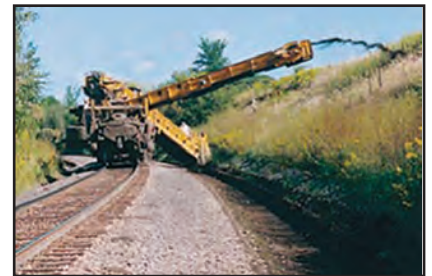
Swinging boom. The machine can excavate on either side of the track - without "Y" ing the machine.
