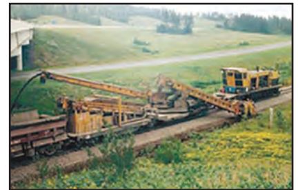
Conveyor. The Badger's conveyor system discharges material on either side of the track or into an air dump car towed behind.
